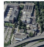
Waste water treatment plant
