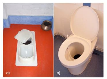
Figure 3: a) a urine-diverting dry squat toilet from India (photo: S.Vishwanath <u>www.rainwaterclub.org</u>); b) a urine–diverting dry toilet from Sweden (photo: Dana Cordell).
