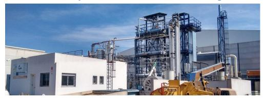
Ingelia has announced a commercial Hydrothermal Carbonization (HTC) in Tuscany, Italy, which will process 80 000 ton/year of sewage sludge. The plant, developed and designed by Ingelia for major Italian water service company ACEA, in Chiusi, Tuscany, will transform sewage sludge into biolignite (fuel) and a biofertiliser. Ingelia is already operating two
