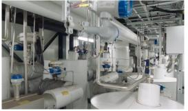
OxyPower HTC<sup>™</sup> simplifies both nitrogen and phosphorus recovery. Nitrogen is extracted from the separated nitrogen-rich wet oxidized process water by ammonia stripping. Up to 60% of the nitrogen in the sludge is separated as ammonium sulphate.
