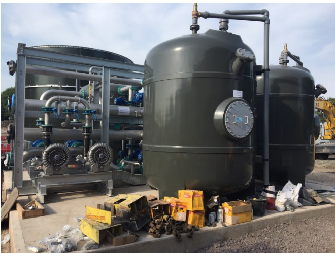
Photos above: Severn Trent Water. Top: CoMag (Finham wwtp). Middle: Nereda. Below: Filter Clear (Codsall wwtp).
