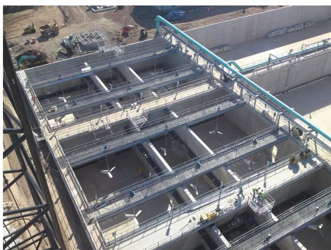
New-build biological P-removal (EBPR) capacity at Severn Trent's Minworth wwtp (near Birmingham), today treating c. 1.8 million p.e. with EBPR.
